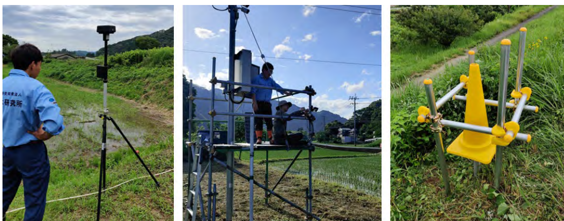
Figure 2. Tracking deformation using RTK (left); Adjusting the CCTV cameras (middle); Maintaining the piezometers (right).
