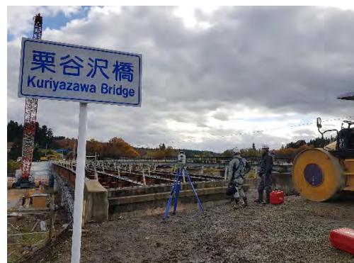
Bridge construction site.
